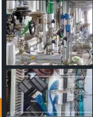
Installation, pre-commission and commissioning for instrumentation equipment
